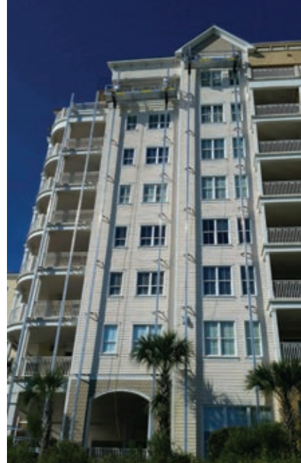
A ReechCraft PowerMast climbs a beachfront building in the U.S. to clean windows.
