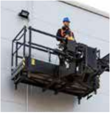
Man platform ready
