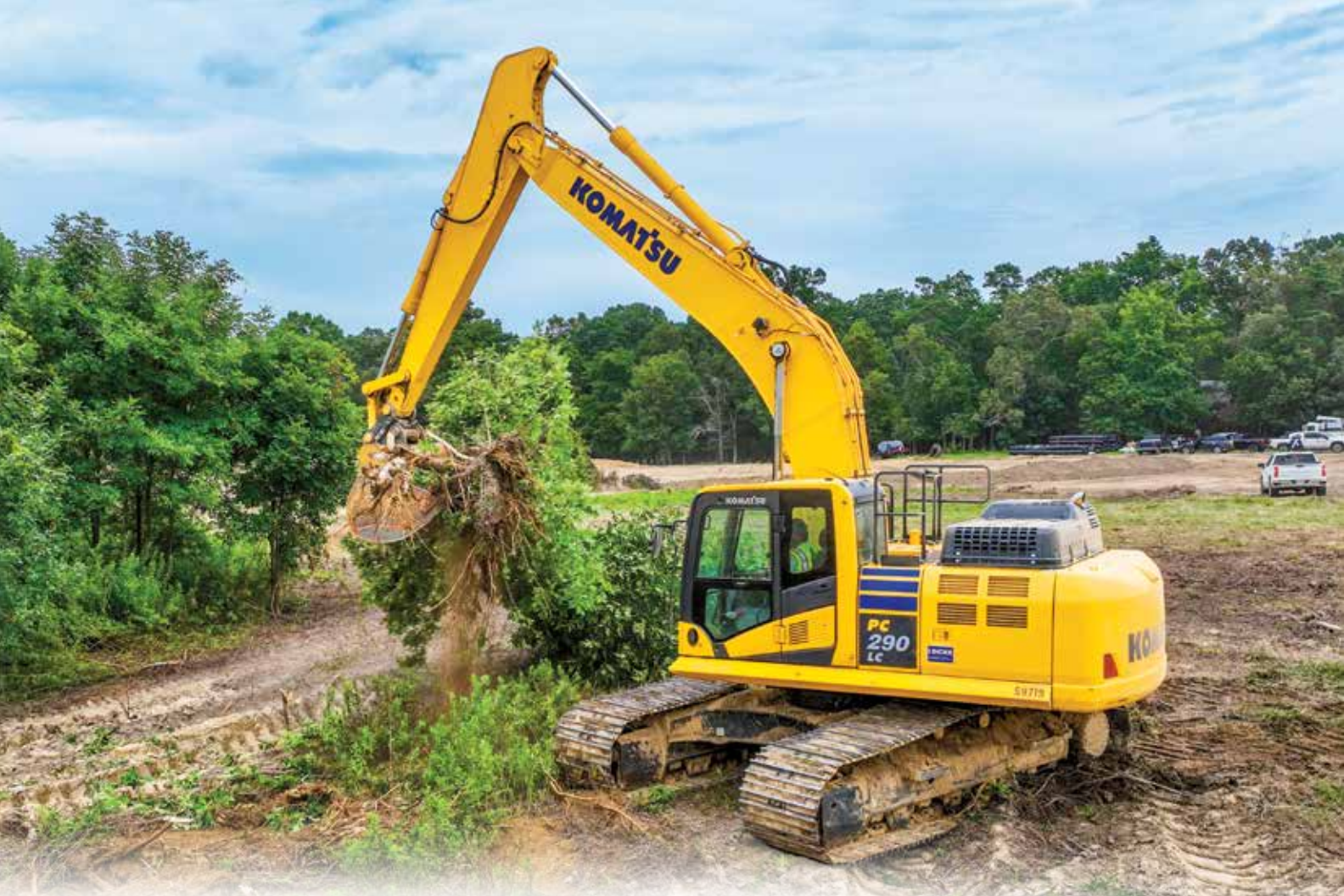
An operator clears brush with a Komatsu PC290LC excavator.
