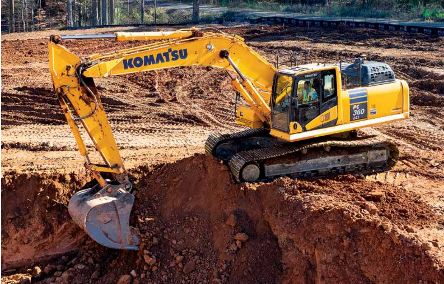
An operator cuts to grade on a bench with a Komatsu PC360LCi-11 IMC excavator. "With IMC, everything is done in a lot faster and smoother manner," said GPS Technician Joey Keller.
