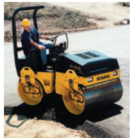
BW135AD in action on asphalt
