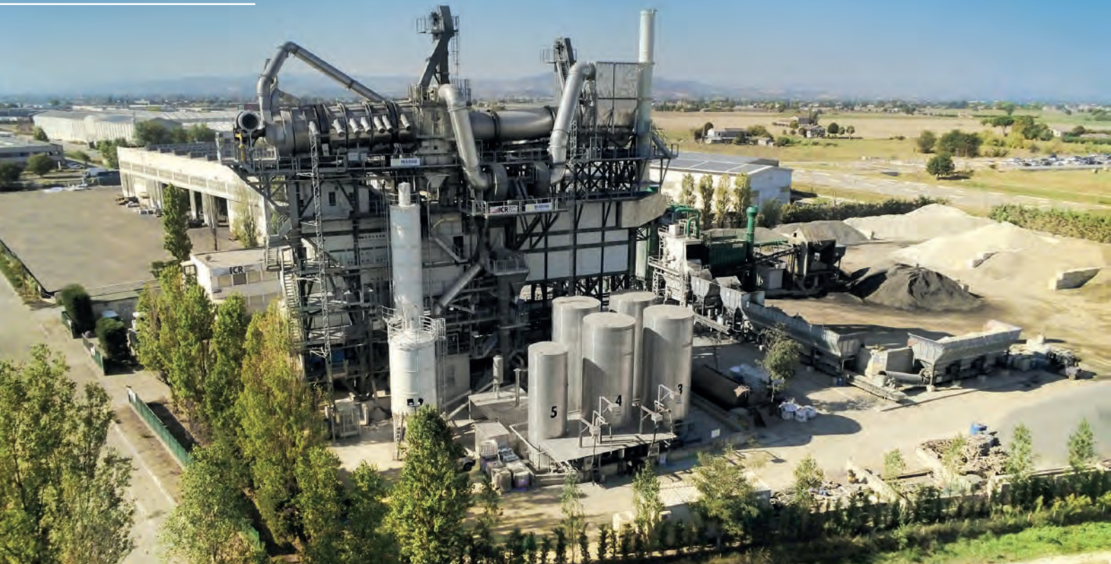
Marini Master Tower, Cesena (Italy)
