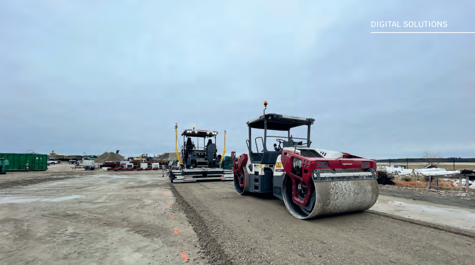
Jobsite at Houston International Airport
