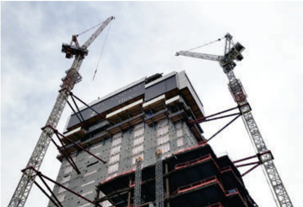
Cranes tower over CIBC Square, a $3 billion development on Bay Street in Toronto.
