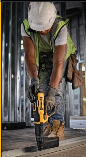
› Interior commercial framing
