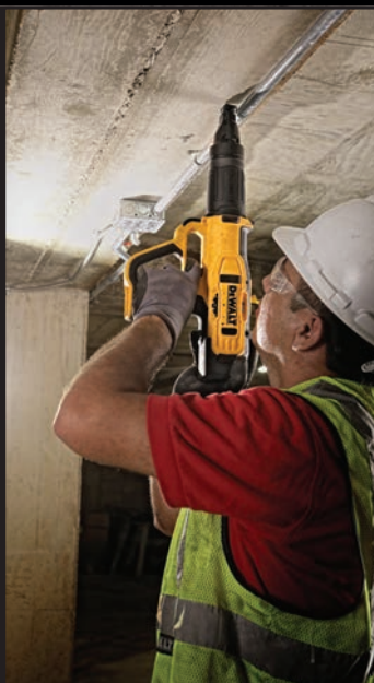
› Mechanical, electrical, and plumbing installations
