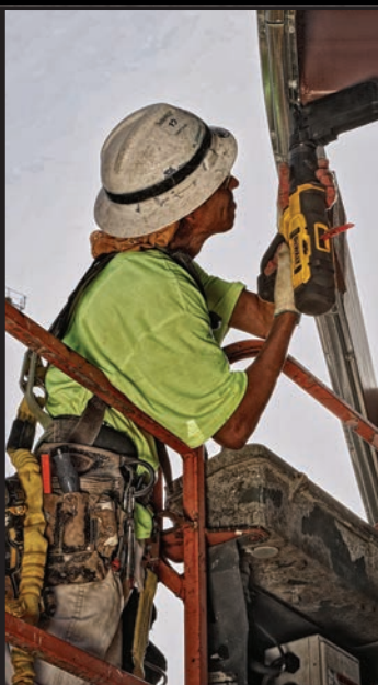
› Light gauge steel installations
