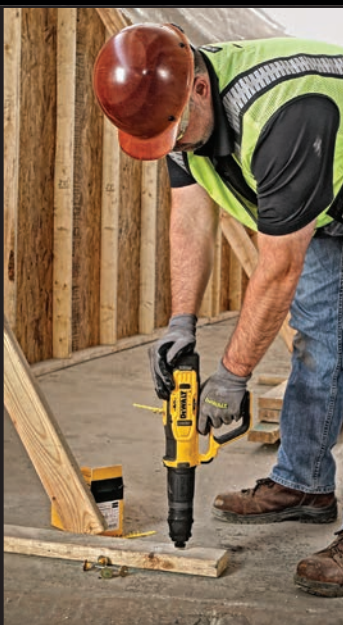
› Formwork and wood installations
