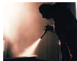
Surface Preparation Protective Coating Application
