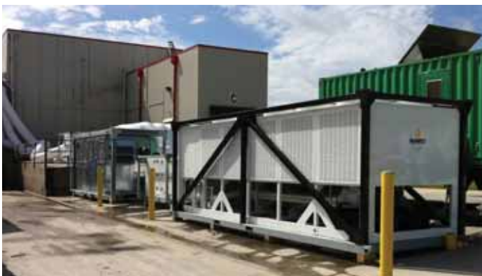
150 Ton Portable Air Cooled Chiller Package
