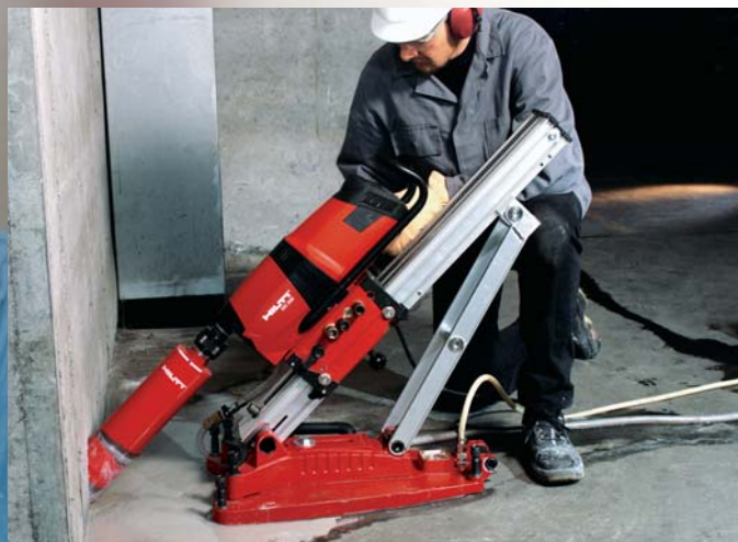
Versatility: Drilling at an angle for gas pipes
