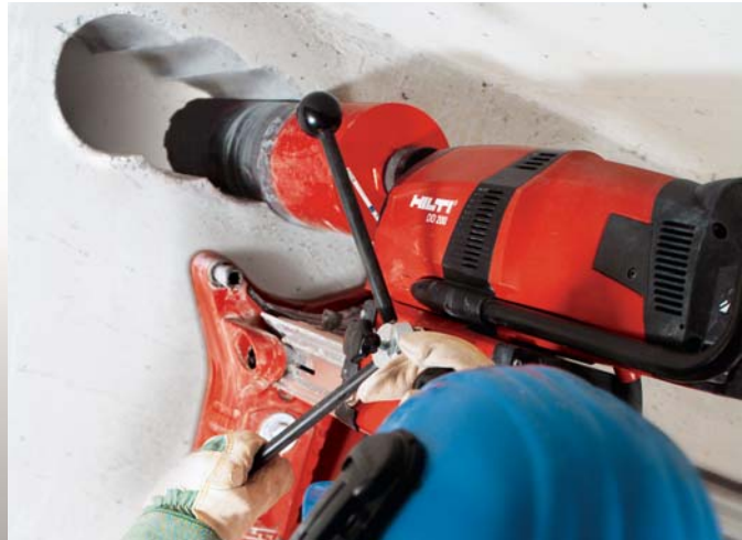
Stitch drilling: Openings for cable trays
