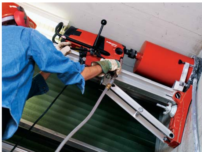
Coring for air-conditioning ducts - with maximum stability
