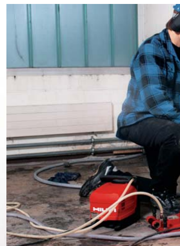
Top coring efficiency in plumbing installation
