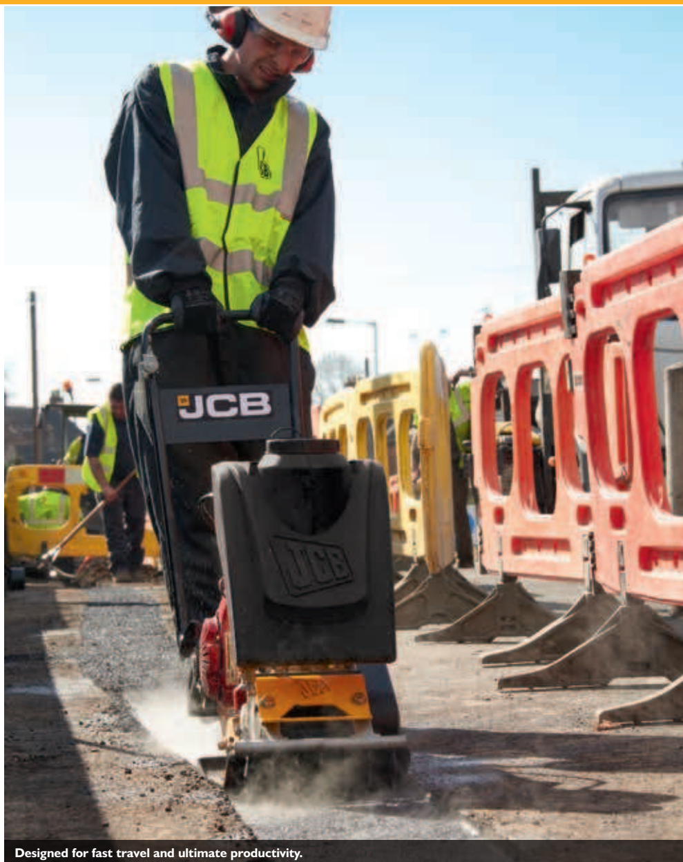
Low vibration levels for improved operator comfort.
