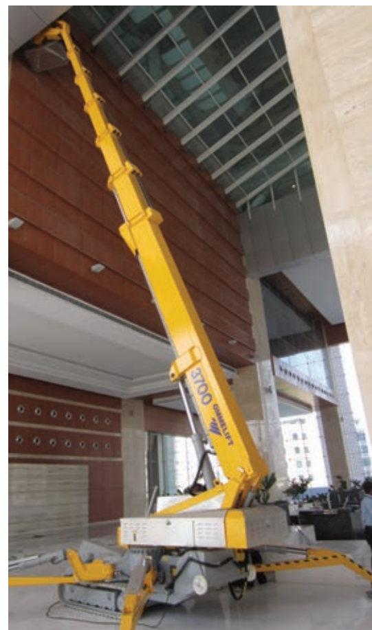
An Omme Lift tracked platform owned by Mtandt carrying out maintenance work.
