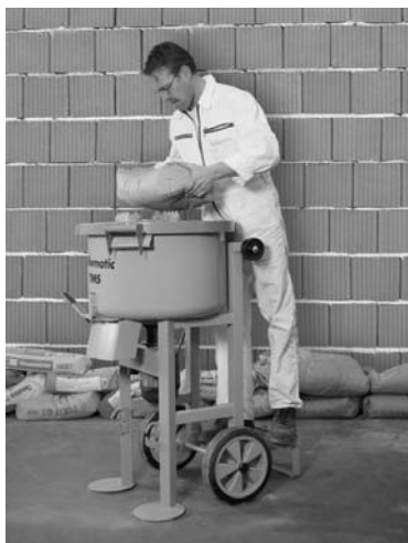
Figure 3. Filling Mixing Tub
