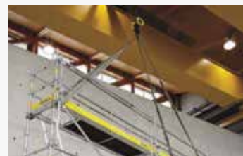
Quick repositioning by crane or guide roller
