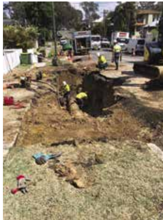
Trench safety is crucial
