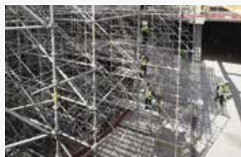
Secure erection workflow thanks to pre-defined connection points on the rosette
