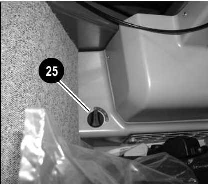
Fig. 69: Air conditioning rotary switch
