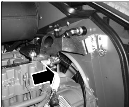
Fig. 127: Cleaning the oil cooler
